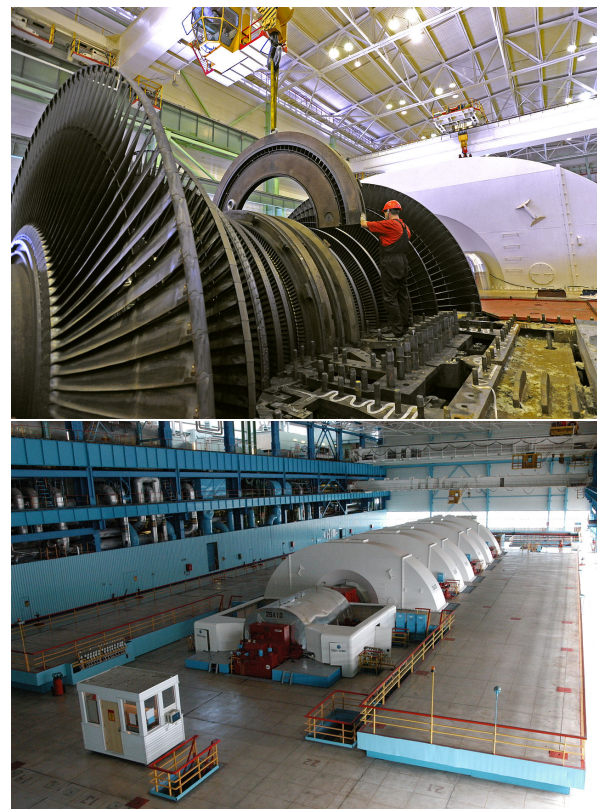
Figure 5.34: One of the turbines at the Russian Balakovo nuclear power station (~1 GW plant power), in maintenance (top) and during installation (bottom).
