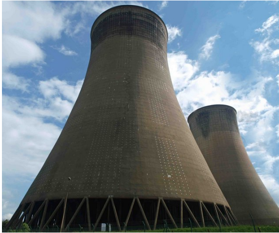
Figure 9.9: Cooling towers of the Eggborough coal power plant (1967, 1960 MW) in the United Kingdom. In these towers, the heat extracted from the water in the condenser is dissipated into the atmosphere. This cooling is done through a secondary water circuit, which is brought into contact with the atmosphere and partially evaporates.
