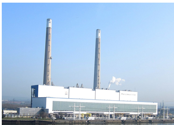
Figure 9.27: The Porcheville power plant, running on coal until 1987, then on oil until 2017, when it closed down. It mainly served peak demands.
