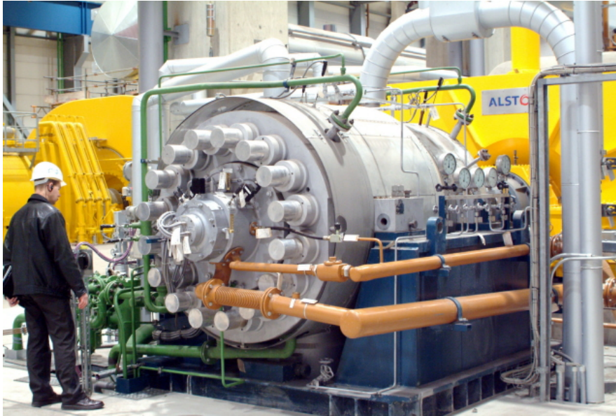
Figure 9.2: A pump from the manufacturer KSB delivering 2500 t/h of water at 350 bar in a steam power plant. Liquid pumps are usually powered by an electric motor, but this model is mechanically driven by the turbine and must therefore operate over a wider speed range. Its maximum power is 38 MW; the power of the driven turbine exceeds 800 MW.
